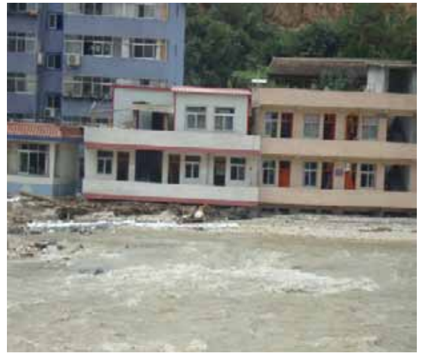
Heavy rains filled the Bailong River, causing devastating mudslides.
