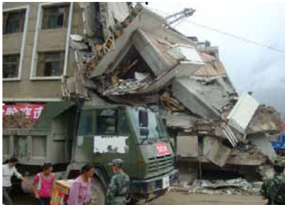
Homes and buildings collapsed.
